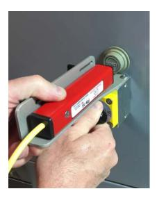
**STEP 4** – At this point the actuator should be firmly attached to the switchgear door with the plunger tip over your button.
