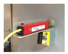
The magnet should be firmly against the switchgear door. If the magnet is not set firmly against the door, it will likely not have enough holding power to stay on the door when actuated.
