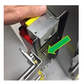
Additionally, the magnet used to hold the ABL3 actuator on the MCC door could present a pinch hazard. To prevent an injury the follow procedures should be followed:
